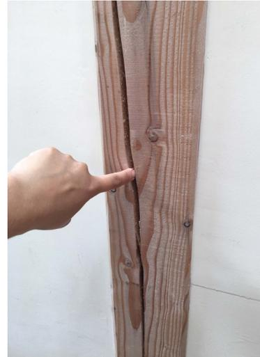
Larch is one of the most durable of the softwoods and is the contractors choice for any post that needs to go into the ground due to its longevity and natural resistance to rot and fungus. However, although larch is the most durable, it is also likely to crack more and release more sap than spruce or other mixed softwood posts (which will also crack).
