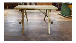
Fix the 2 diagonal pieces to the underside of the table top and to the A frame leg on each side using the 50mm wood screws. NB. There are two pencil marks on the inside of the A frame to help guide placing.
